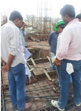
*Inspecting steel connections before pouring concrete can be approved*
