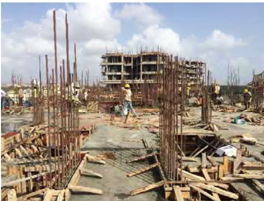
Concrete slab and column preparation
