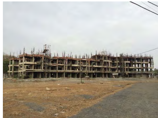
Residential high-rise construction
