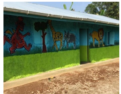
PDI Education Center newly renovated by the Lehigh team
