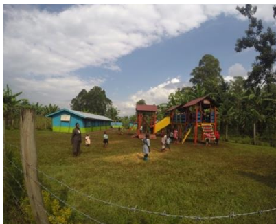
Completed school renovation and playground build. August 2015
