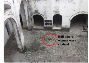
Pictures taken for the report on the structures of the slave castles.
