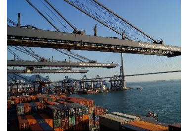
A quay crane at Terminal 4 in Hong Kong
