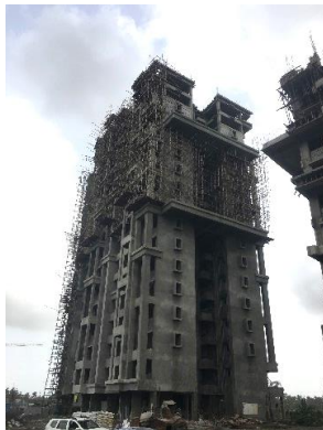
Visit to Viva City Construction Site
